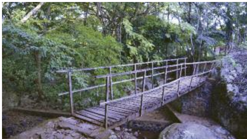
Bridge crossing the Mulunguzi River in Zomba Botanic Garden. (BGCI)
