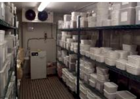
The seed bank of BHP Billiton Iron Ore contains seeds for use in mine site restoration. The room is maintained at 15°C and 15% relative humidity. (Brad Stokes)
